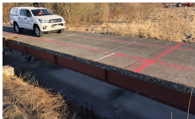
FIGURE 2. Test Bridge UniBw M (Alexander Mendler, 2022)
